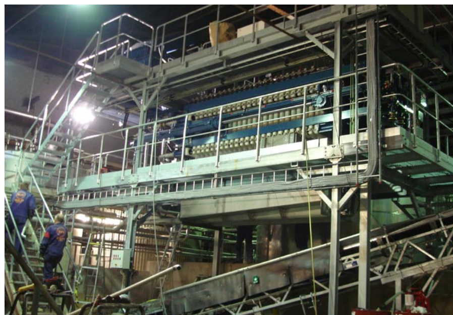
In the second filtration stage, the lignin is washed with acidic water, pressed and formed into solid fuel.
